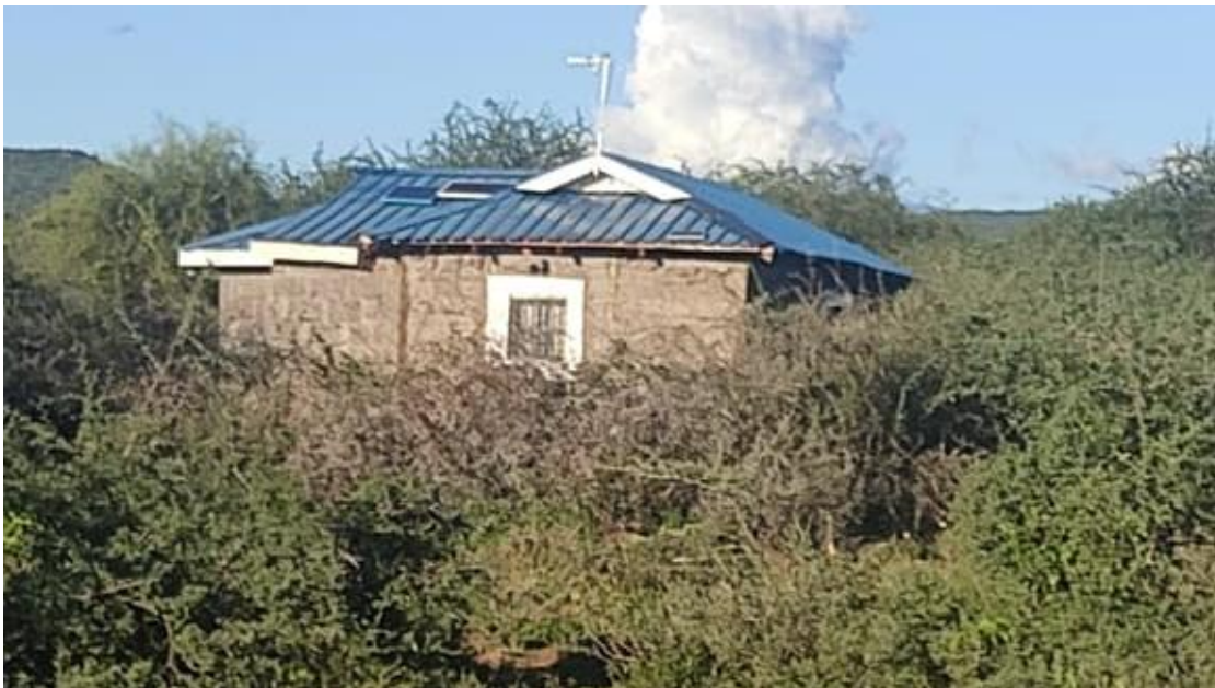
A stone walled house fitted with a solar panel
