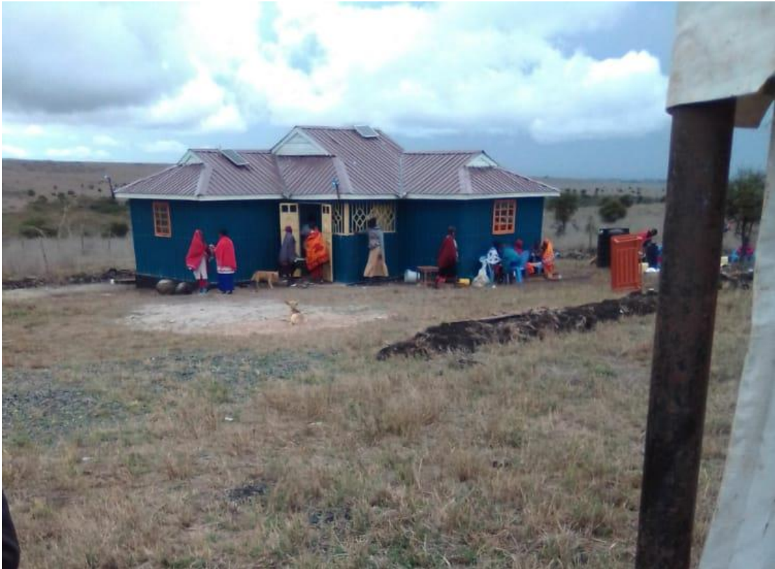
A modern Maasai house made of iron sheets and fitted with a solar panel
